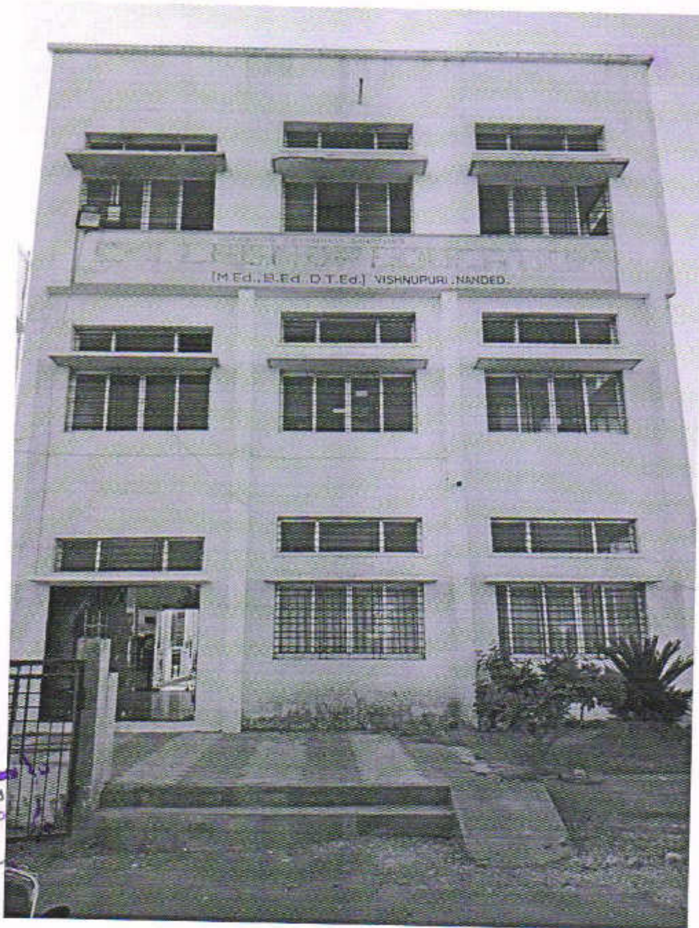
Rear view of the building
