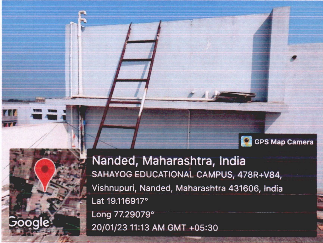
Constructed Water Harvesting Tank ( capacity 20000 Ltr)
